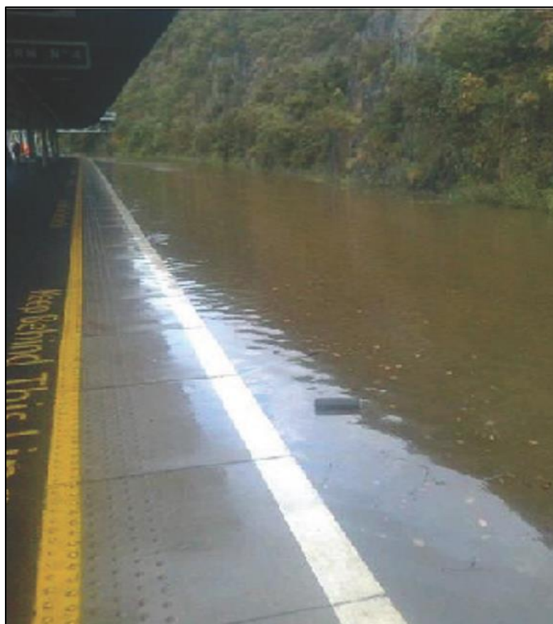
Plate 2.9 Flooding at Plunkett Station on the 17 th of October 2012
