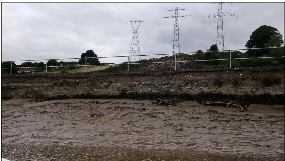
Plate 2.2 Typical condition of the wall/shoreline between Ch.340 and Ch.1090 (Photo taken at approx. Ch.650)
